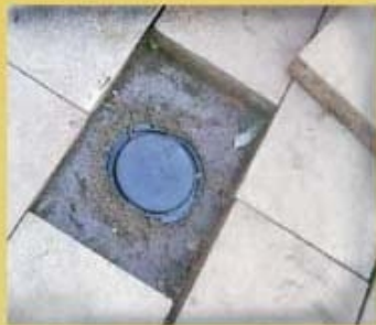
Installation under pavers
